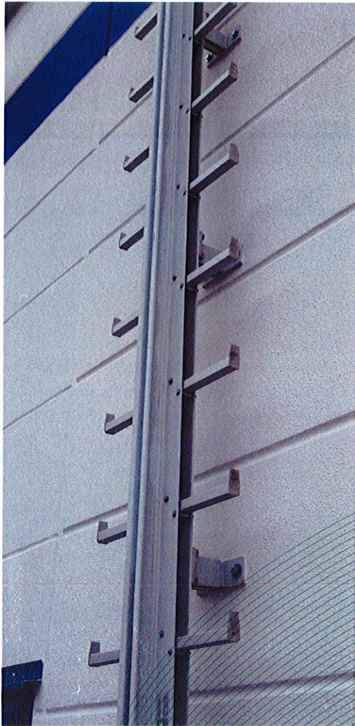
Fig. 8: Single stile ladder with foldable sprouds Fig. 9: Single stile ladder with lashing straps
